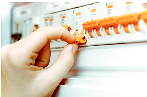
Figure: Contrary to the fuse, the circuit breaker does not need to be replaced with a new unit once open. The contacts may be reclosed using a reset lever
